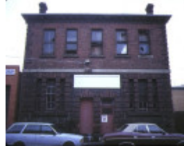
former grosvenor common school bond street collingwood front view jun1985
