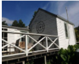
Formerly detached rear kitchen (now bathroom)
