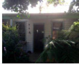
Entrance to north cottage
