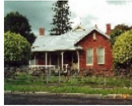
Toora Post Office residence (2000)
