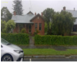
Toora Post Office Residence
