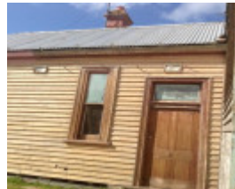
North side doorway
