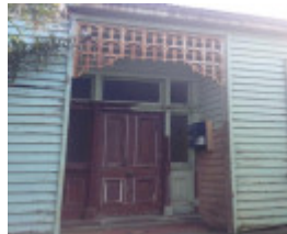
Residential entrance on south side
