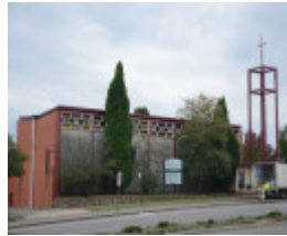
All Saints (former Christ Church) Mitcham, south elevation, 2012.JPG
