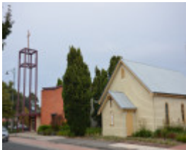
All Saints (former Christ Church) Mitcham, view of former church and 1958 church from north east, 2012.JPG
