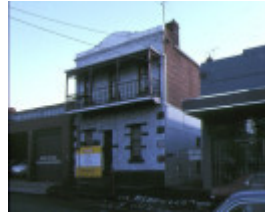
1 Belmont Johnston Street Collingwood front view
