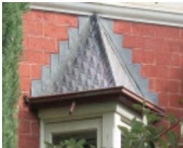
1 Maitland Street Glen Iris
