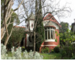
1 Maitland Street Glen Iris
