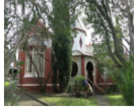
1 Maitland Street Glen Iris
