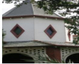
1 Maitland Street Glen Iris
