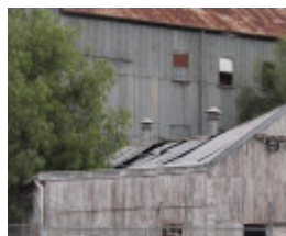
H1011 FORMER WIMMERA FLOUR MILL AND SILO COMPLEX LHA 2015 6.JPG
