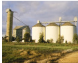
1 former wimmera flour mill & silo complex gibson street rpanyup silos side view
