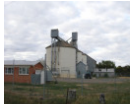
FORMER WIMMERA FLOUR MILL AND SILO COMPLEX SOHE 2008
