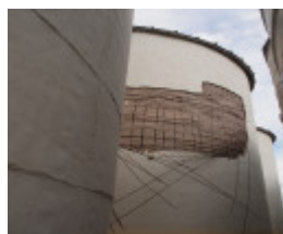
H1011 FORMER WIMMERA FLOUR MILL AND SILO COMPLEX LHA 2015 9.JPG
