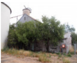
H1011 FORMER WIMMERA FLOUR MILL AND SILO COMPLEX LHA 2015 4.JPG
