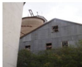
H1011 FORMER WIMMERA FLOUR MILL AND SILO COMPLEX LHA 2015 5.JPG
