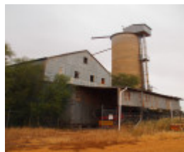
H1011 FORMER WIMMERA FLOUR MILL AND SILO COMPLEX LHA 2015 3.JPG
