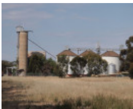
H1011 FORMER WIMMERA FLOUR MILL AND SILO COMPLEX LHA 2015 1.JPG
