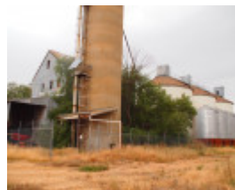
H1011 FORMER WIMMERA FLOUR MILL AND SILO COMPLEX LHA 2015 2.JPG
