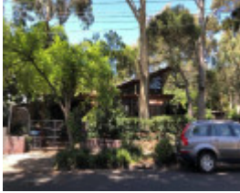
16 & 16A Glyndebourne Avenue, Toorka
