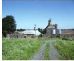
1 former distillery old melbourne road dunnstown property view
