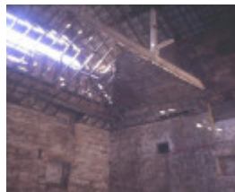
former brinds distillery old melbourne road dunnstown roof main building she project 2003
