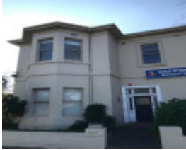
1219-1225 Dandenong Road, Malvern East
