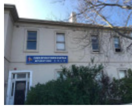
1219-1225 Dandenong Road, Malvern East
