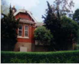
FORMER LODGE, AUSTIN HOSPITAL
