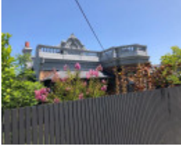
50 Stanhope Street, Malvern
