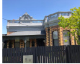
50 Stanhope Street, Malvern
