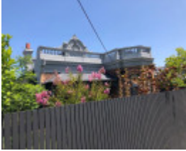
50 Stanhope Street, Malvern
