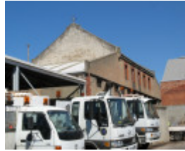
Municipal stables Sth Yarra_north side_18 Feb 08
