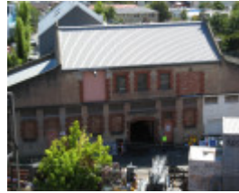
Municipal stables Sth Yarra_south side_18 Feb 08
