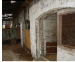
Summer Hill large cow shed west side KJ 10 July 07 65
