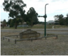
Stand pipe and horse trough, junction of Ross Creek - Haddon Road and School Road, Haddon
