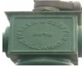
Detail of Standpipe Haddon
