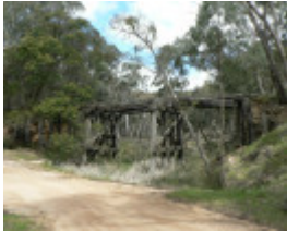
Mt Misery Creek Trestle Bridge, Berringa
