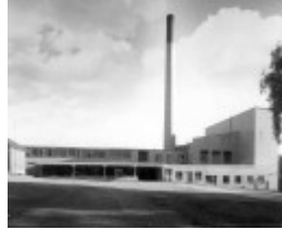
Boiler House and Laundry 1956
