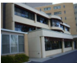
John Lindell Rehabilitation Unit 1999
