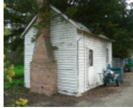
Linton Park Linton Mannibadar Rd Linton, laundry at rear.
