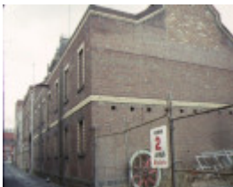
former yorkshire brewery wellington street collingwood rear view
