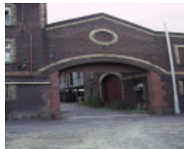
former yorkshire brewery wellington street collingwood entrance to stables
