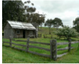
Naringal Slab Hut
