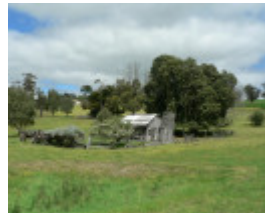
Naringal Slab Hut
