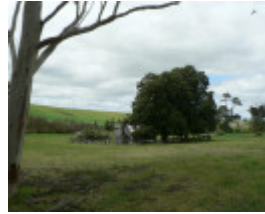
Naringal Slab Hut
