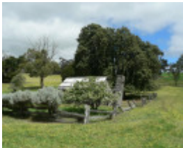
Naringal Slab Hut
