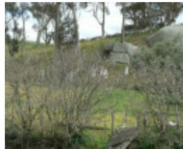
Naringal Slab Hut
