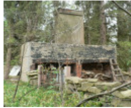
31709 Lawson's Hotel Cambridge St former kitchen chimney 374
