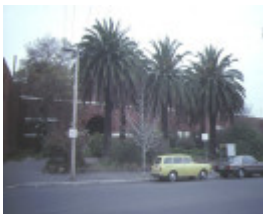
auburn railway station complex garden detail jun1984
