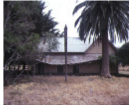
monomeith homestead cranbourne rear view feb1985
