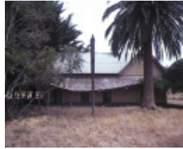
monomeith homestead cranbourne rear view feb1985
