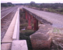
rail bridge creswick creek top view may1995
