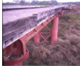
rail bridge creswick creek siding detail may1995
