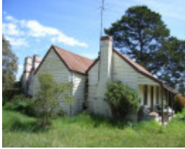
204539 11 Argyle Road, Argyle
