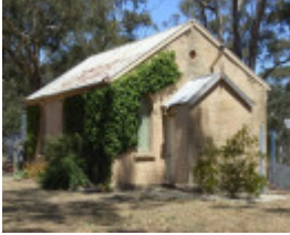
Wesleyan Church (former), 204623 1 McClellans Crescent, Argyle
