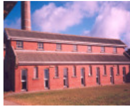
H02030 point nepean bathhouse2
