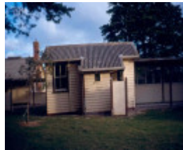
H02030 point nepean isolation hospital
