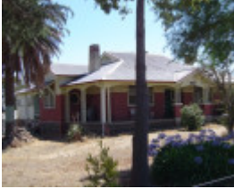
215715 381 Axedale Kimbolton Road, Axedale
