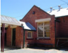
196709 Axedale Primary School No 1008, 81 High Street, Axedale
