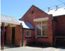
196709 Axedale Primary School No 1008, 81 High Street, Axedale
