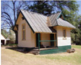
2270 Mclvor Highway, Axedale Marydale outbuildings
