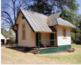
2270 Mclvor Highway, Axedale Marydale outbuildings
