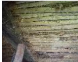
192577_Emu Creek_Red Tank Road_197_img10
