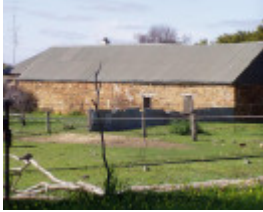
192577_Emu Creek_Red Tank Road_197_img01
