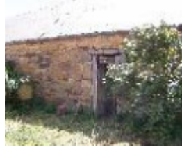
192577_Emu Creek_Red Tank Road_197_img04
