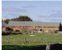
192577_Emu Creek_Red Tank Road_197_img08
