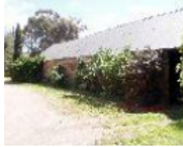
192577_Emu Creek_Red Tank Road_197_img03
