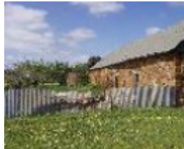
192577_Emu Creek_Red Tank Road_197_img07
