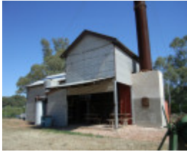
LOCK NINE PUMPING STATION SOHE 2008
