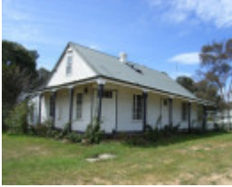
203611_Heathcote_Northern Highway South_6360_img01
