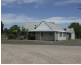
216164_Knowsley_Knowsley- Eppalock Road_011_img01
