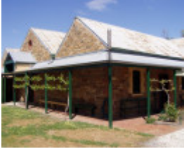
219301_Mandurang South Road_303 img 01
