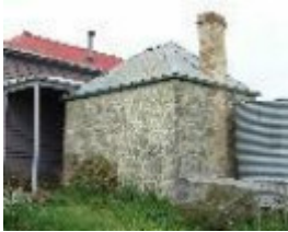
206184_Redesdale_Kyneton Redesdale Road_2351 img09
