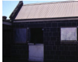
stables 1875 lara homestead derrinallum entrance
