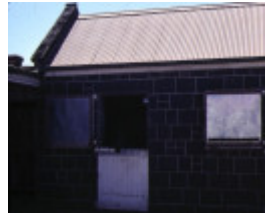
stables 1875 lara homestead derrinallum entrance
