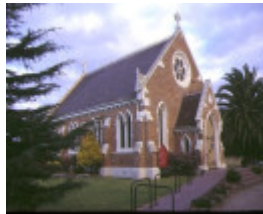
1 christ church old dandenong road dingley village front view
