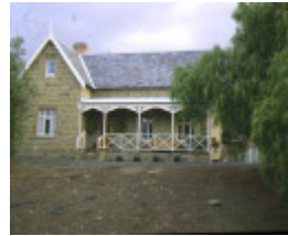
1 holy trinity anglican church merrawarp road ceres vicarage front view
