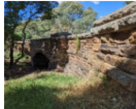
Bridge viewed from the approach looking north (?)
