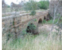
1 bridge over hughes creek avenel nov 99
