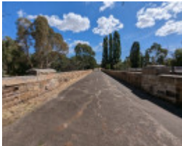
View from centre of bridge looking west
