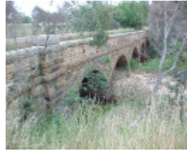
1 bridge over hughes creek avenel nov 99
