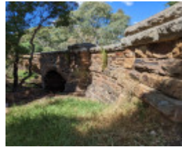
Bridge viewed from the approach looking north (?)
