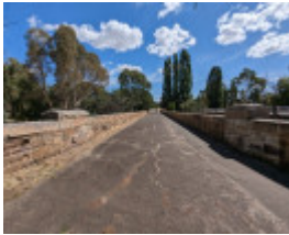
View from centre of bridge looking west
