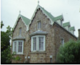
1 coriyule homestead drysdale side view of homestead
