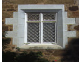
coriyule homestead mcdermott road drysdale detail of stone framed window
