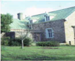
coriyule homestead mcdermott road drysdale view of top floor
