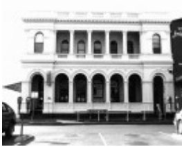
Sandhurst Savings Bank, Hargreaves Street
