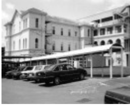
Bendigo Goldfields Hospital, Lucan Street
