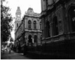
Bendigo Post Office, 51-67 and 69 Pall Mall
