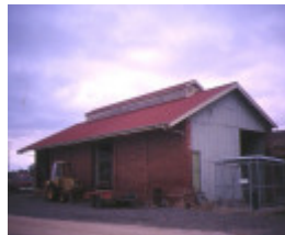
dunolly railway station goods shed may1995
