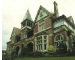
1 north park woodland street essendon front view sep1996
