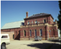
court house town hall dunolly side view
