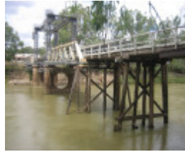
Tooleybuc Bridge_Piangil_Feb 2008_mz_Victorian Approach Spans
