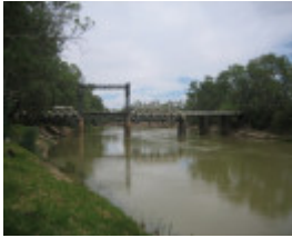
Tooleybuc Bridge_Piangil_Feb 2008_mz_West Elevation
