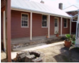
H2169 RIMG0148 - c.1849 cottage, 15-19 Gawler street, portland
