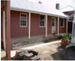
H2169 RIMG0148 - c.1849 cottage, 15-19 Gawler street, portland
